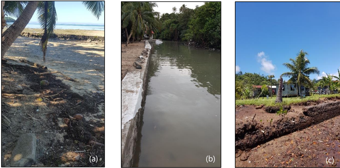
Figure 2.2 Examples of seawalls built in rural Fijian communities to protect village infrastructure and reduce erosion (a) Narikoso, Ono Island, Fiji (Source: Author, 2019). (b) Under construction at Vabea, Ono Island, Fiji (Source: Author, 2019). (c) Navunievu, Vanua Levu, Fiji (Source: Author, 2018).
